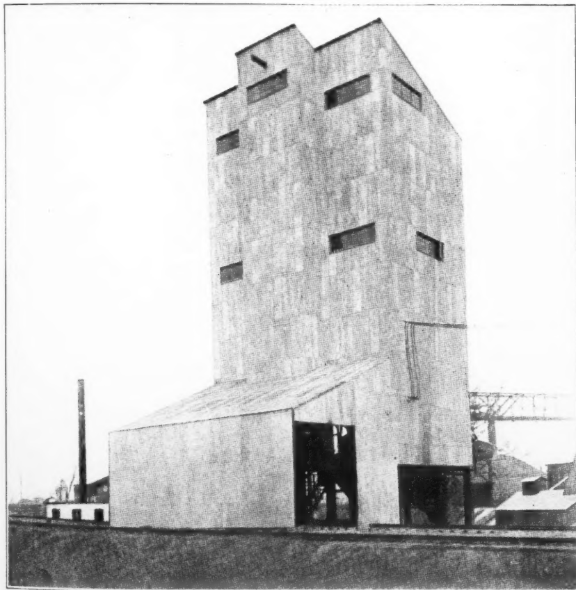
Note the High Track Where the Slag Is Dumped Into the Crusher Hopper
